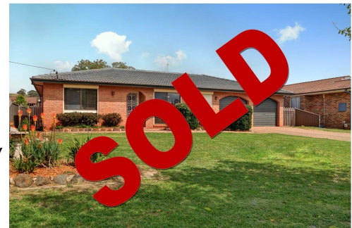
62 Dalley Street, Goulburn
